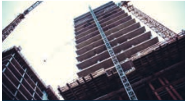
Earthquake resistant Seismic Zone Level V Design
